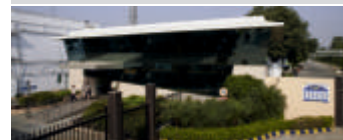
Taper Roller Plant
