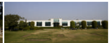
Taper Roller Plant
