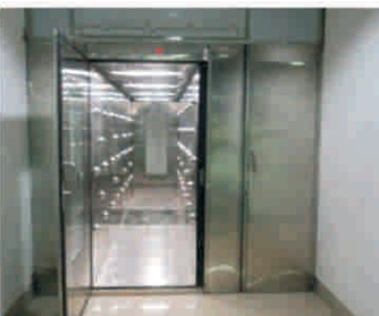
Single point entry into Manufacturing Area by walk through air shower to prevent dust in the manufacturing environment.
