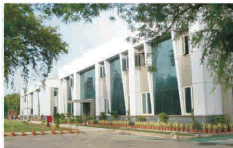
Plant Side View
