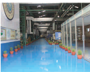
Overview of Plant
